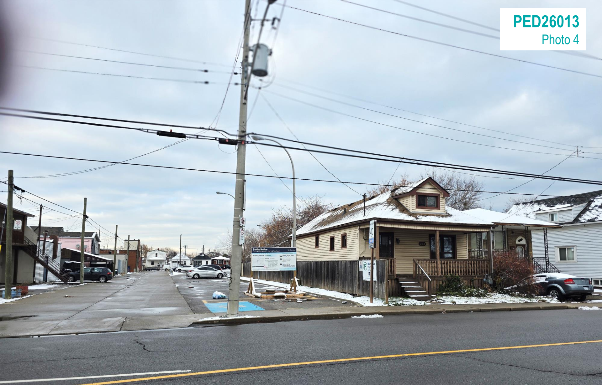
Adjacent property to the east on Britannia Avenue
