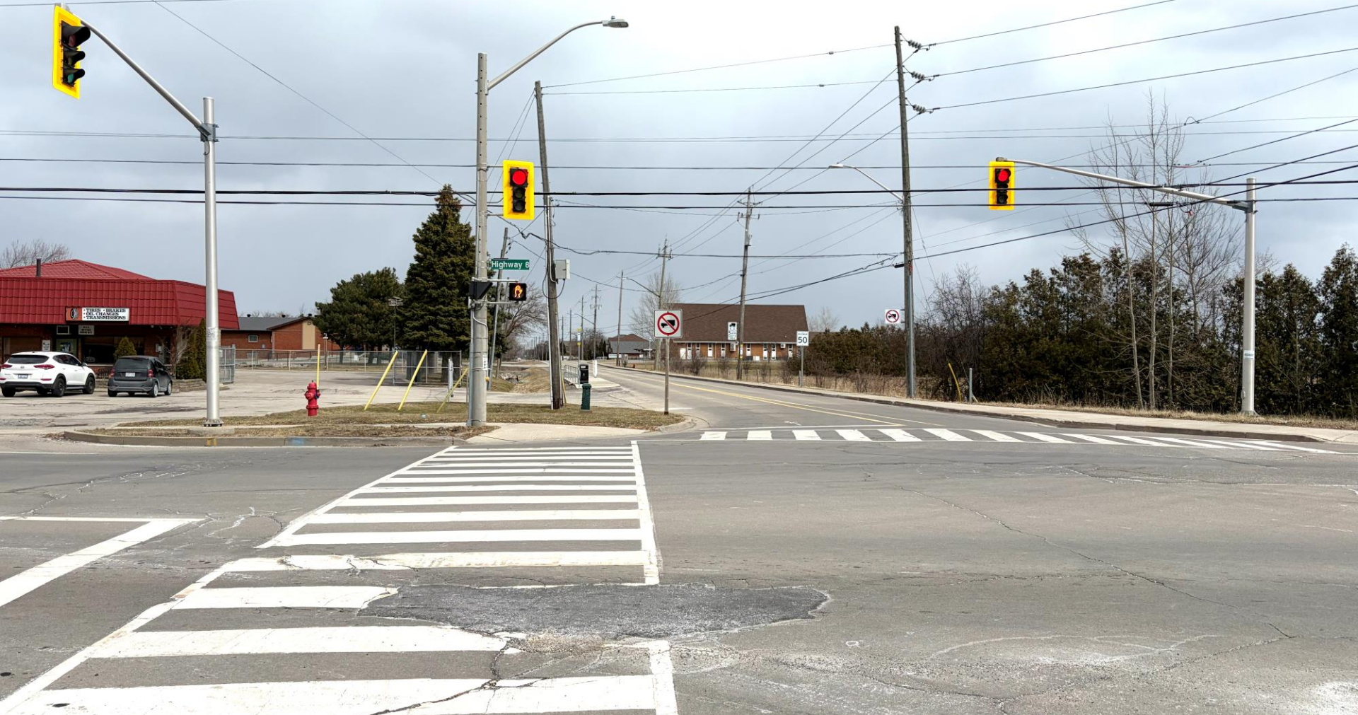
Looking North on Glover at Highway No. 8
