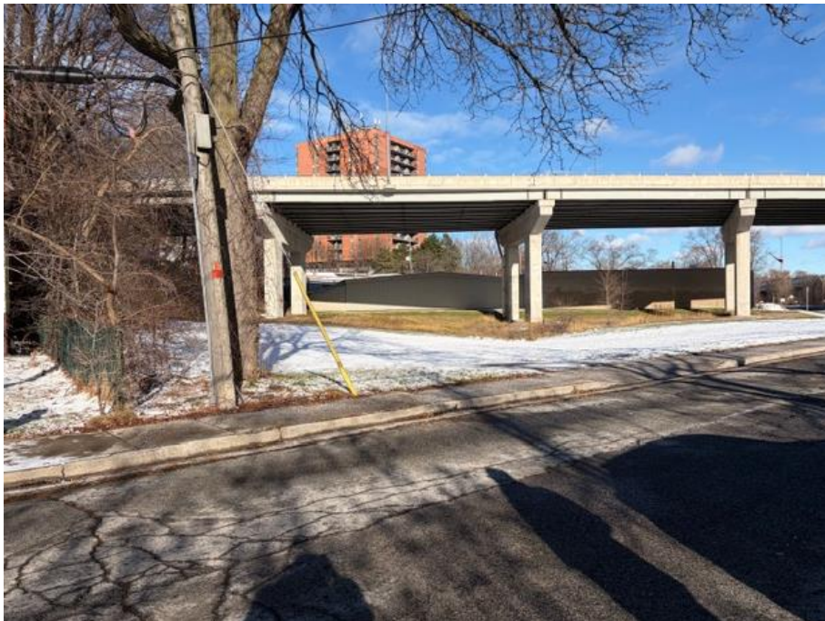
Figure 3 – View of 128 Tope Crescent facing North-East (site visit)
