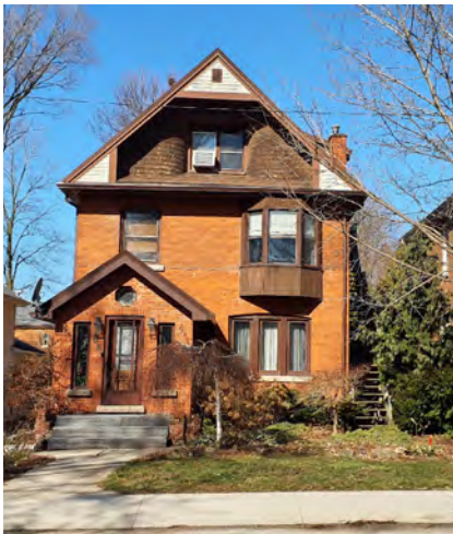
Example of Contributing B Property
