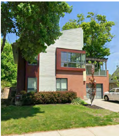
Example of Non-Contributing Property
