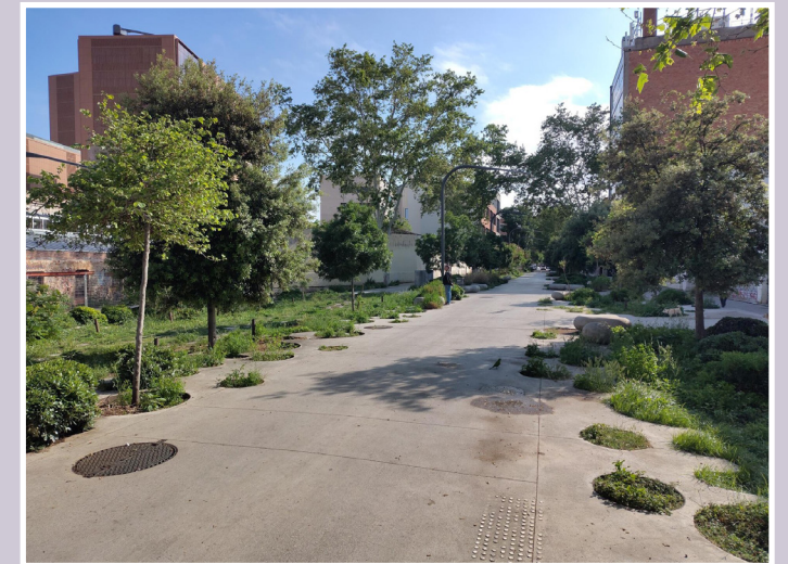
Figure 33- Barcelona. Credit: R Hauschulz
