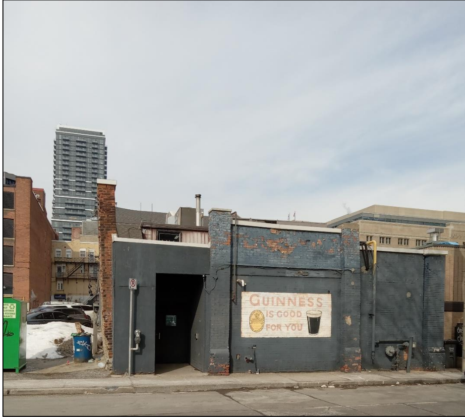
Figure 7: View of rear (east) elevation facing Catharine Street South. (City Staff, March 3, 2026).
