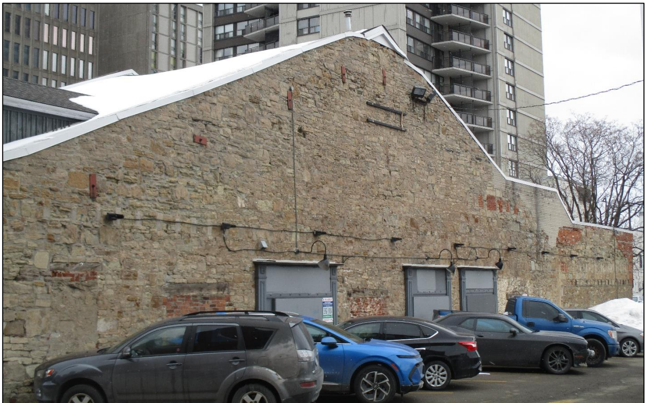
Figure 4: Detail view of side (south) elevation showing masonry construction.
