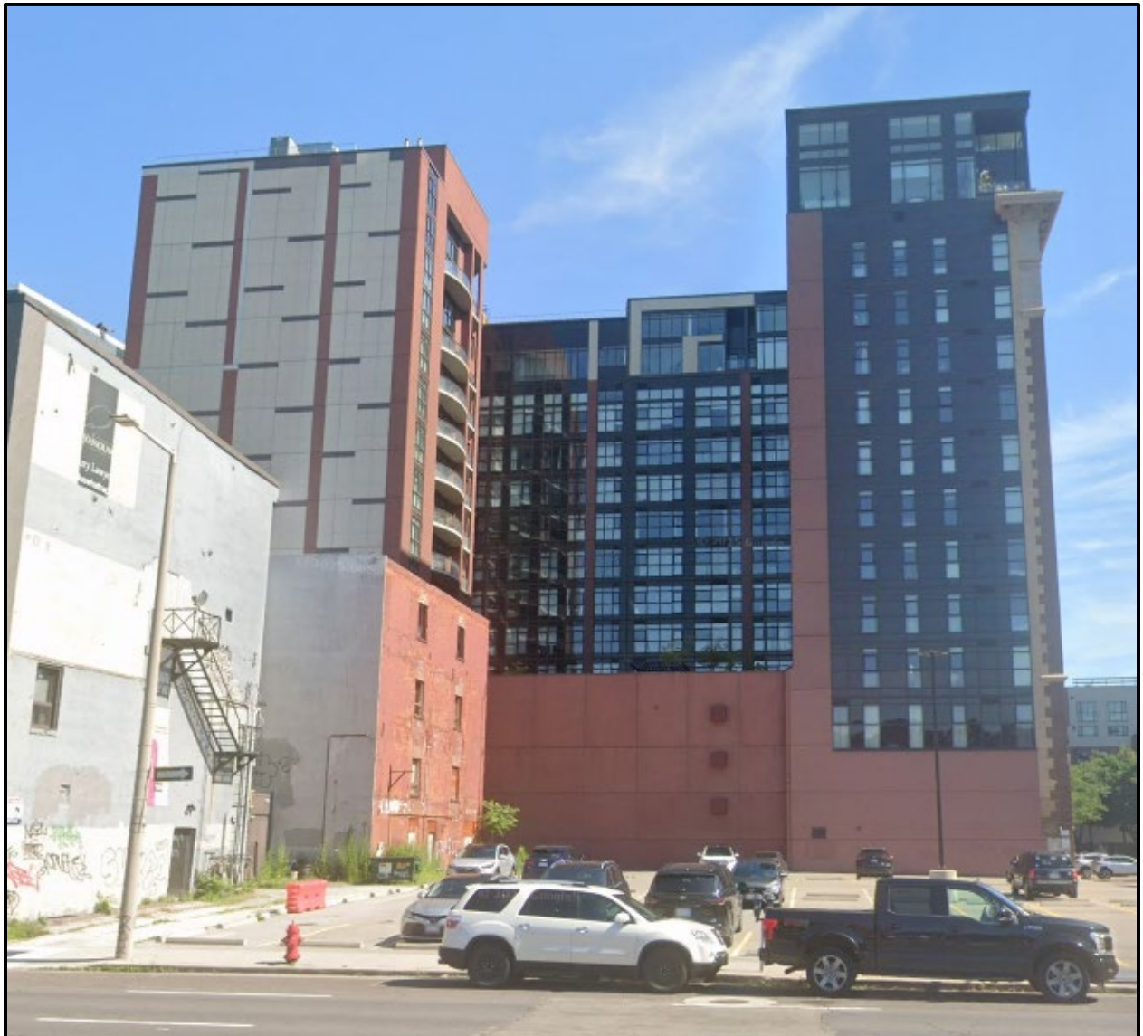
Figure 3: Rear (south) elevation of the Royal Connaught looking north past Main Street East(Google Earth, 2024)
