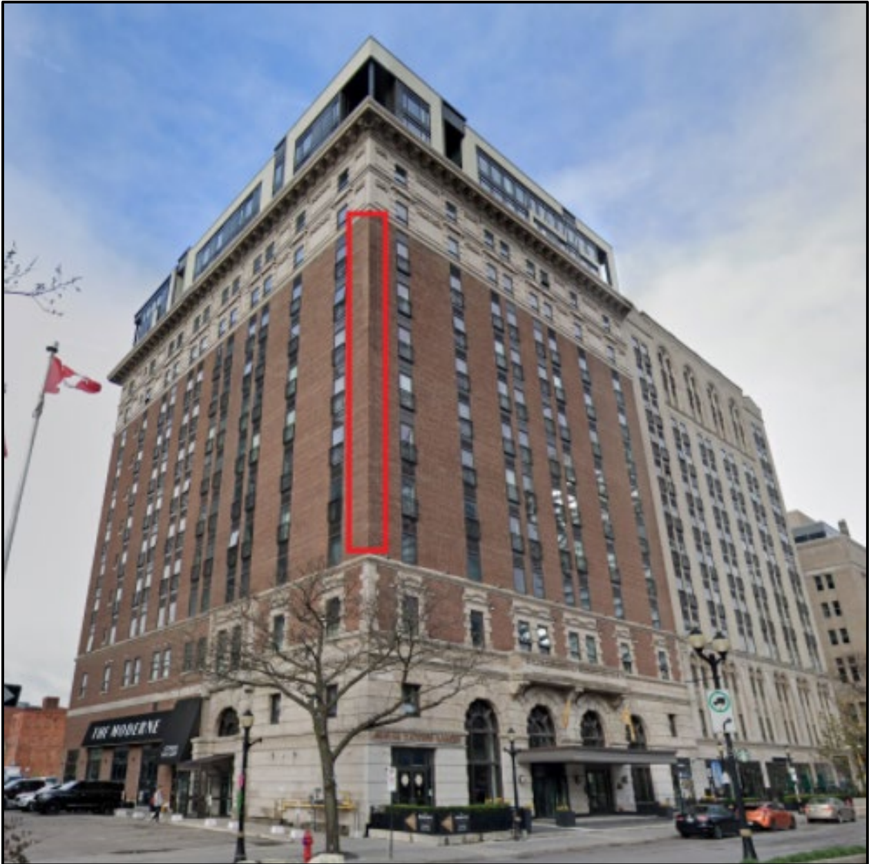
Figure 4: Area of the proposed vertical expansion joint in the northeast corner of the Royal Connaught, outlined in red (Google Earth, 2023)
