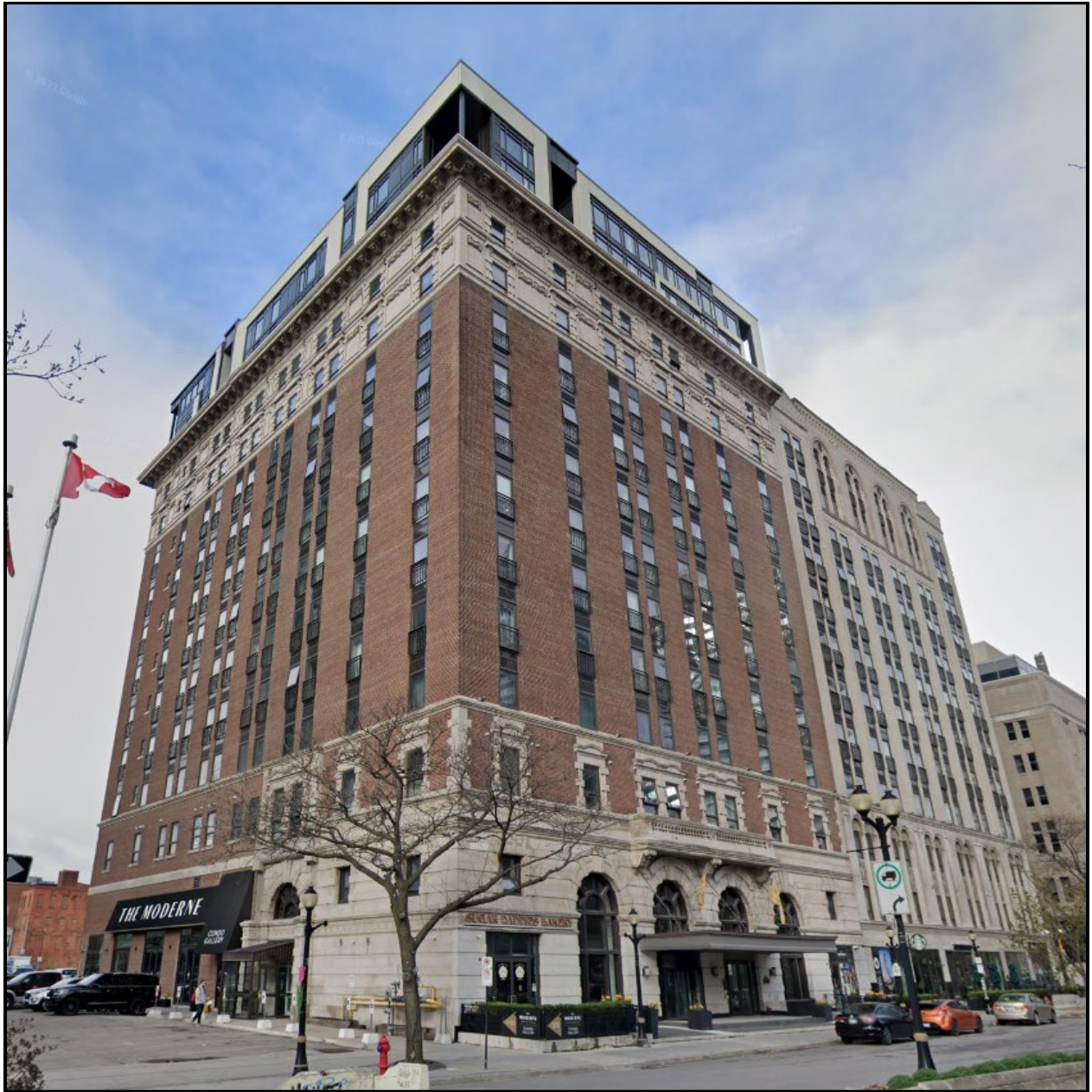
Figure 1: Front (north) and side (east) elevations of the Royal Connaught (Google Earth, 2023)
