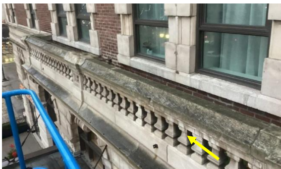
Figure 4: Cast stone cleaning example.
