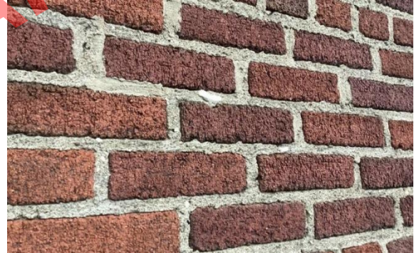
Figure 3: Typical masonry mortar profile overview.
