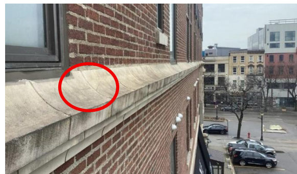
Figure 5: Cast stone crack repair example.
