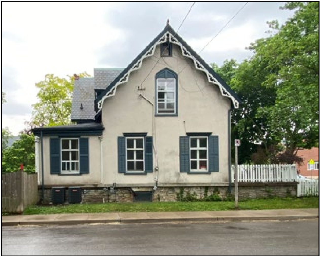
Figure 2: Side (north) elevation from Victoria Street, showing the four windows on this façade that are proposed to be replaced (2023 Site Visit).
