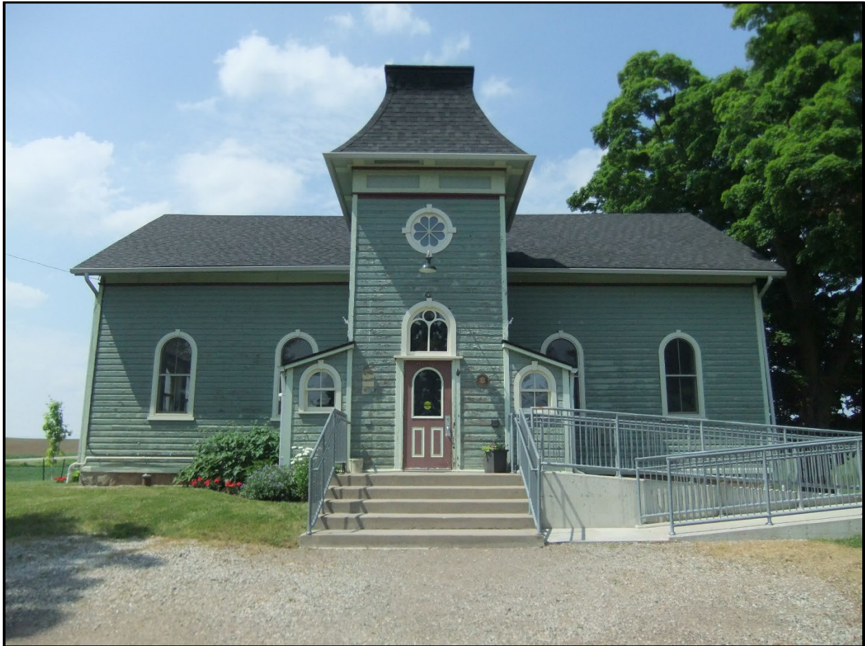
Figure 1: Front (south) elevation of 2295 Troy Road showing the central front tower, accessible entrance and steps (Site Visit, 2024)
