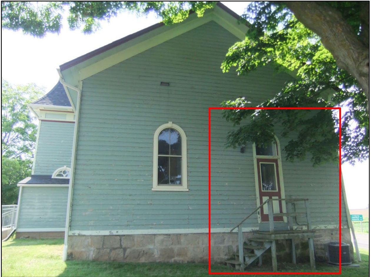
Figure 7: Side (east) elevation of 2295 Troy Road, including area outlined in red for the proposed work to replace the staircase and door, which does not impact heritage features and does not require a heritage permit (Site Visit, 2024)
