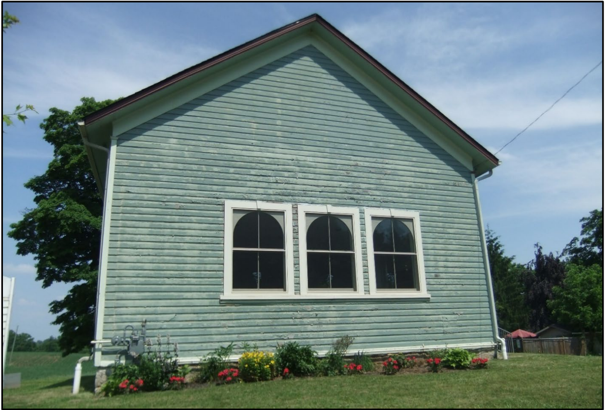
Figure 2: Side (west) elevation of 2295 Troy Road showing the deteriorated wood siding and side gable roof (Site Visit, 2024)
