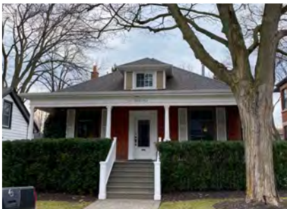
Various roof styles and materials within the HCD
