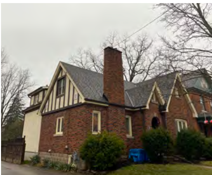
Example of addition located to the side and rear of the main building
