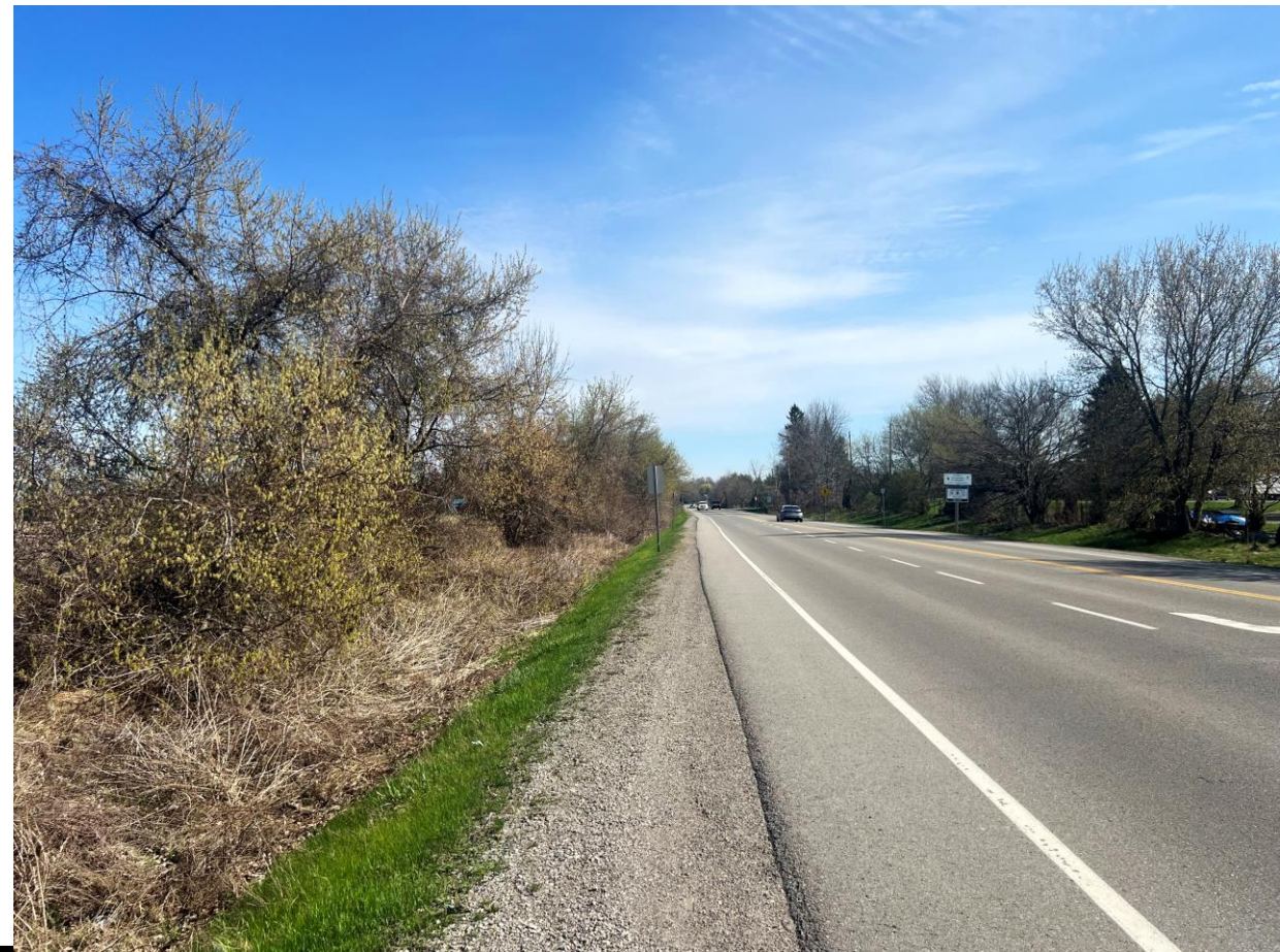
View looking south along Brock Road
