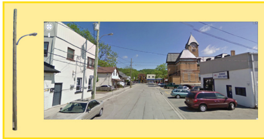
Figure 80 - Cobra Head Lighting on Utility Poles
