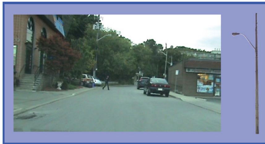
Figure 91 - Davit Style Lighting
