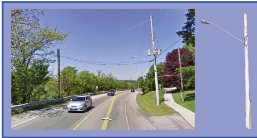
Figure 73 - Cobra Head Lighting on Utility Pole
