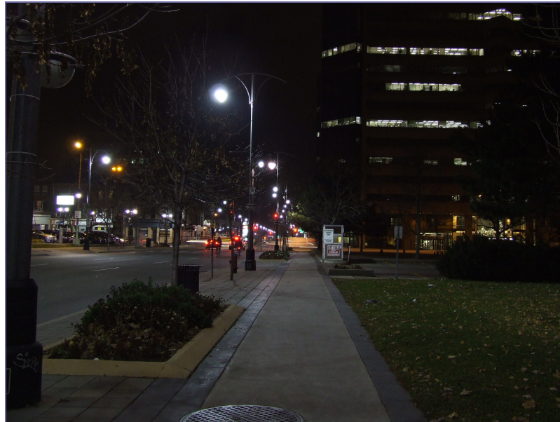
Figure 48 - Overhead Lighting Example
