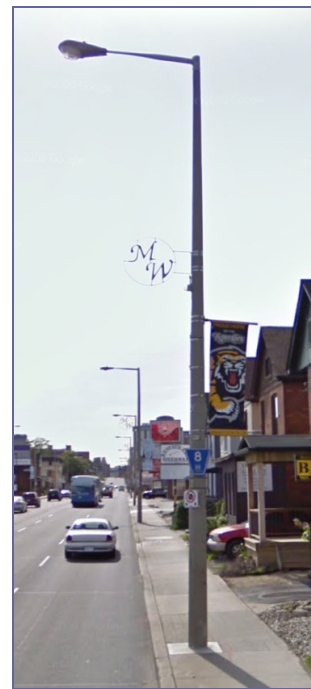
Figure 22 - Examples of Cobra Head Lighting on Poles
