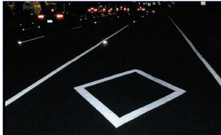
Figure 16 - Retro-Reflective Pavement Markings
