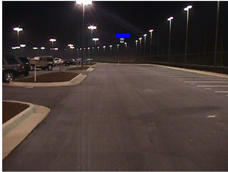
Figure 53 - Open Parking Lot Lighting Example
