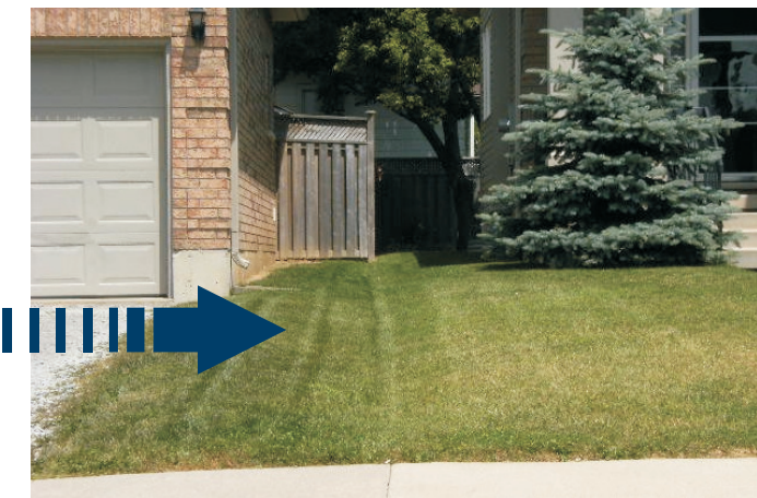
Diagram showing a typical swale design for one-way drainage of a single family residential lot.
