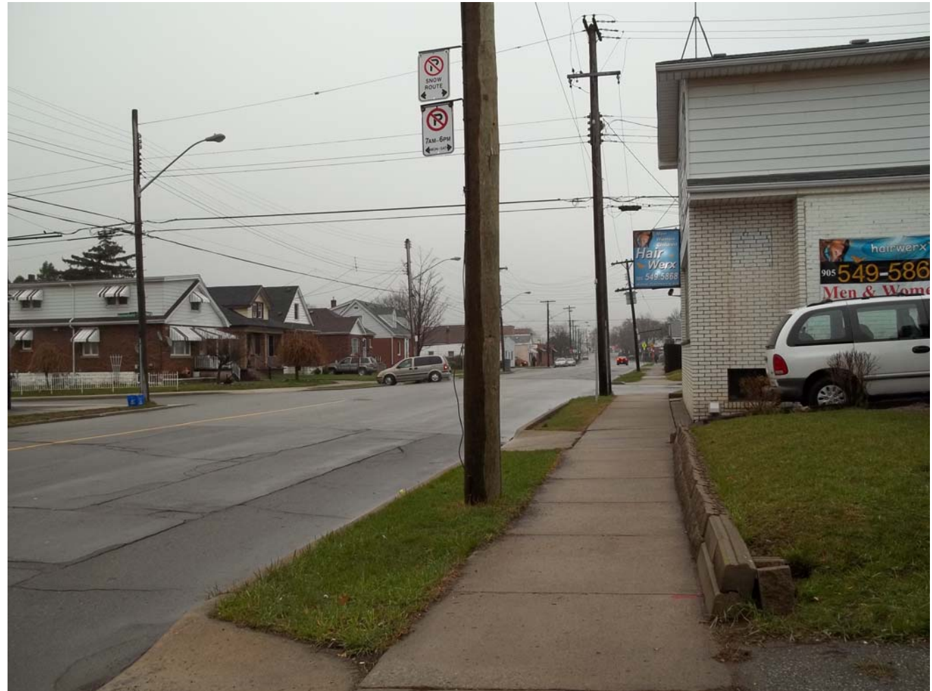
Photo 6 – View from the Northerly access to the East along Main Street
