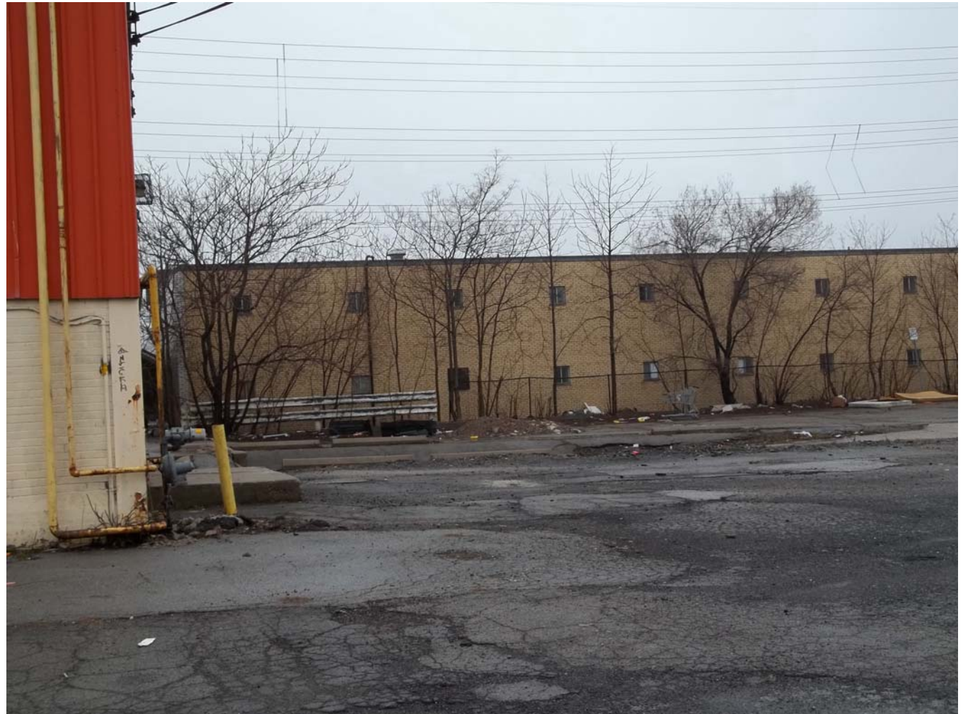
Photo 3 – View from the Subject Lands looking West towards the City Motor Hotel
