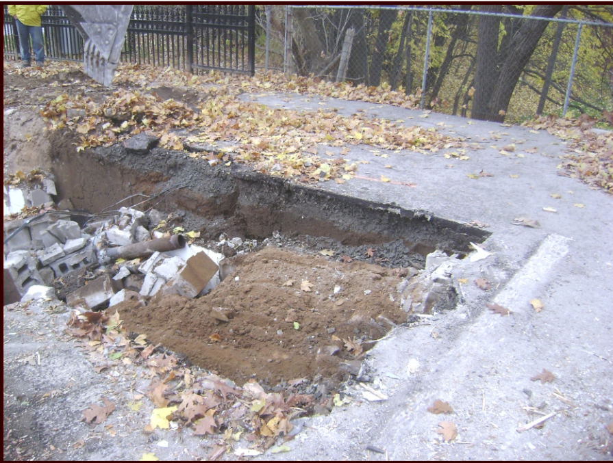
Figure 56: View of Gravel Layer and Fill Soils Beneath Asphalt, Rear of Structure (looking southwest)
