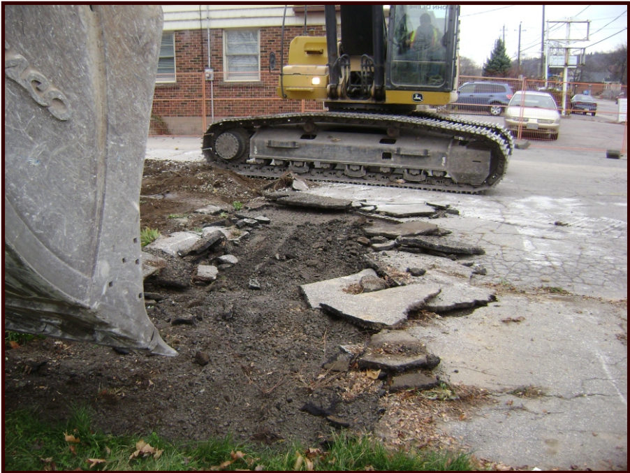
Figure 55: Removal of Asphalt From Around Structure (looking east along front of building footprint)
