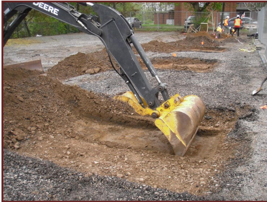
Figure 63: East Boundary Units After Removal of Gravel and Clay Fill (looking north)
