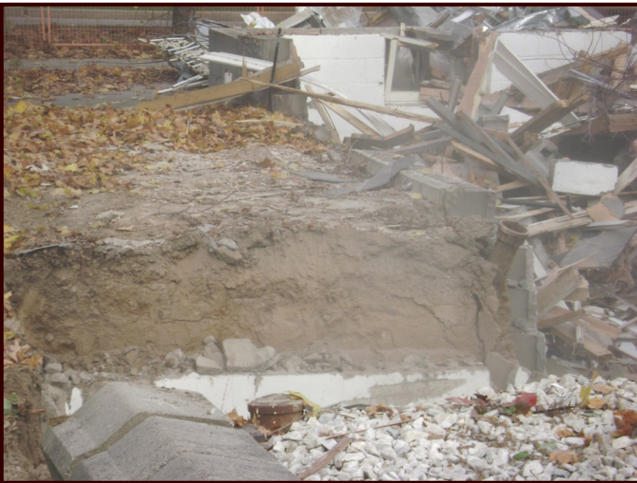
Figure 50: Fill Soils Adjacent to Foundation at Rear of the House (looking north)
