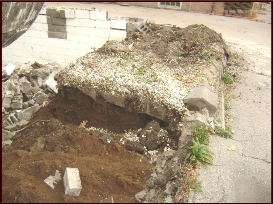
Figure 54: Raised Flower Bed at Front of Structure Containing Topsoil Above Gravel and Geotextile (looking east)
