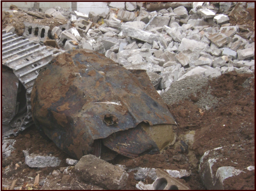
Figure 53: Septic Tank Removed After Pumping
