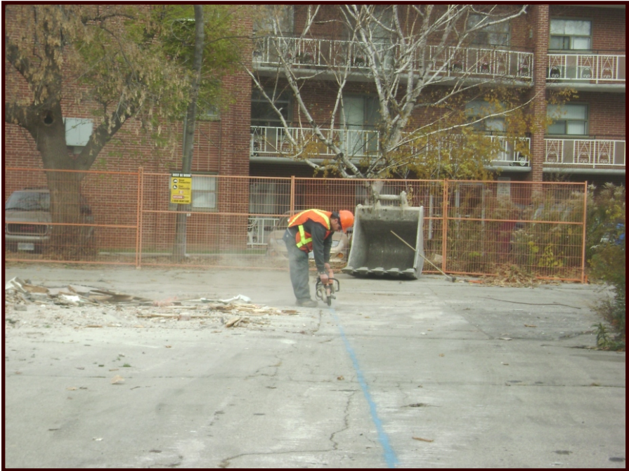
Figure 47: Saw Cutting Asphalt at East Property Boundary (looking north)
