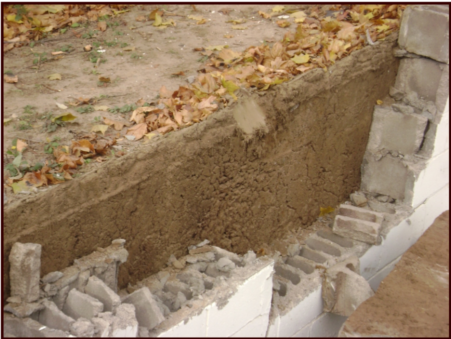
Figure 49: Close Up of Cinder Block Foundation and Intact Fill Soil Beside West Wall of Structure (looking northwest)
