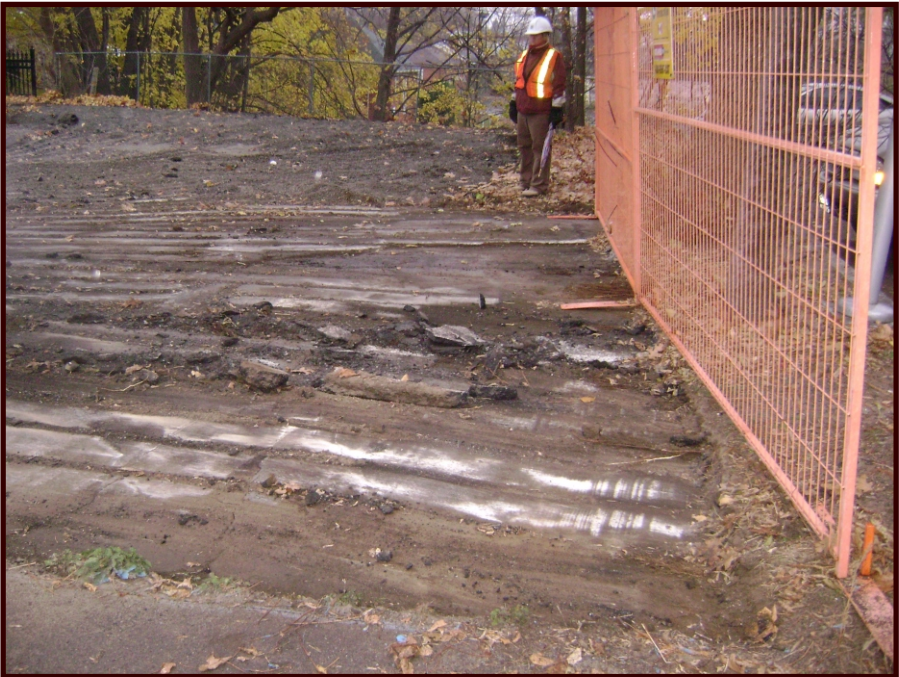
Figure 57: Concrete Slab Beneath Asphalt in Northeast Corner of Property, Extending Beneath Island (looking west)
