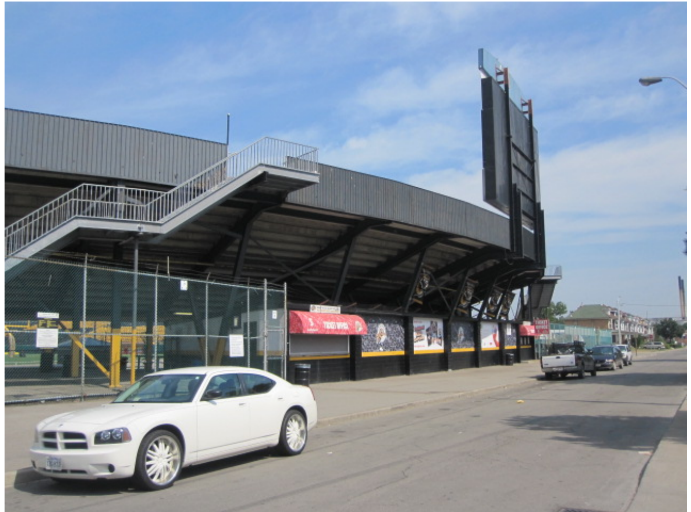
Photo 9 - View of Ivor Wynne Stadium (east stands) from Balsam Ave - East side of the Subject Lands
