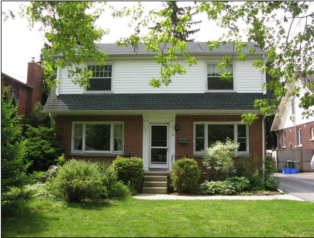
Front (north) façade of the existing house
