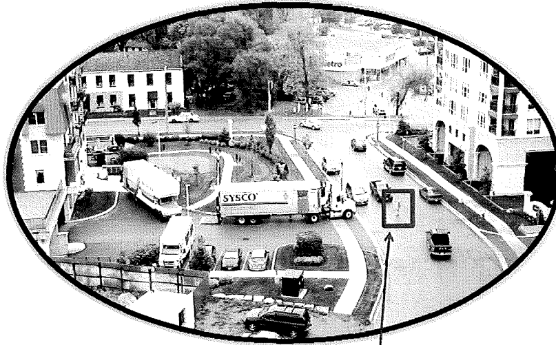
Unfriendly Creekside Drive – Pedestrian forced from sidewalk into the middle of the street.
