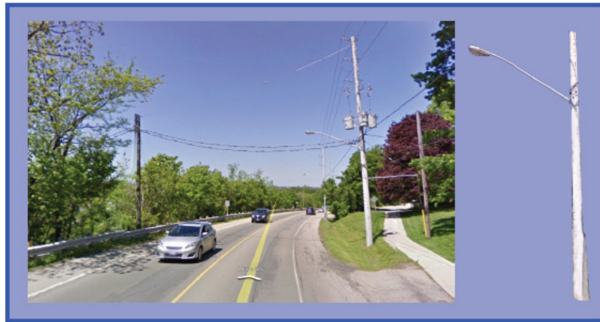
Figure 73 - Cobra Head Lighting on Utility Pole
