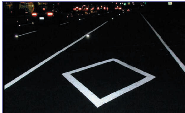
Figure 16 - Retro-Reflective Pavement Markings
