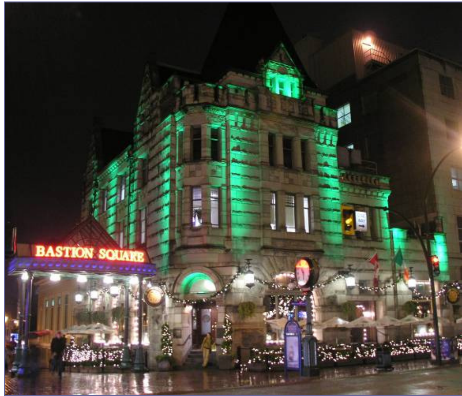
Figure 63 - Colour Changing Lighting
