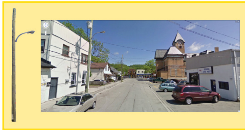
Figure 80 - Cobra Head Lighting on Utility Poles
