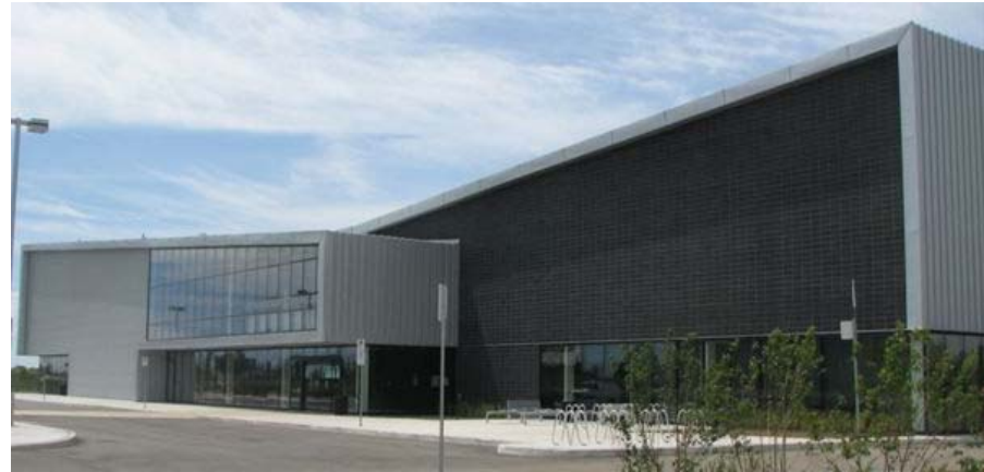
North Wentworth Twin-Pad Arena
