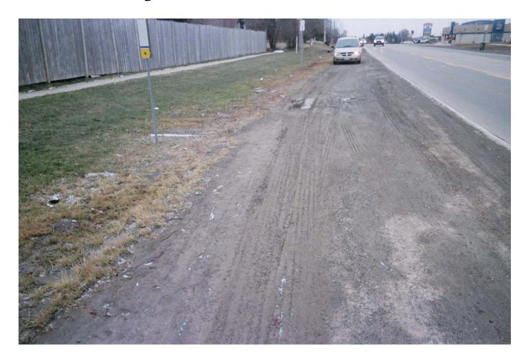
No curb Ramp deploys too steep and into mud and grass
