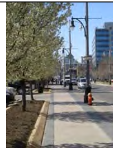
Pedestrian scale lighting along the roadway.
