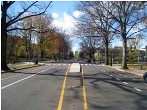
Travel lanes narrowed to create space for a crossing island and bike lanes
