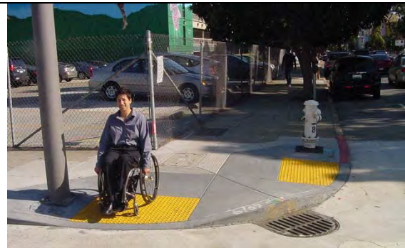
Curb ramps should provide adequate level landing space at the top and bottom of ramp
