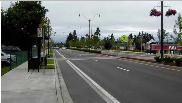
Crossing is placed behind the bus stop and provides a pedestrian refuge for a multi-lane roadway.
