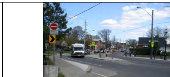
Example of an intermittent median with pedestrian crossing island on a 2-lane road.
