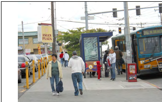
Additional sidewalk on the back side of transit stop allows pedestrians to bypass area where bus boarding/alighting occurs.
