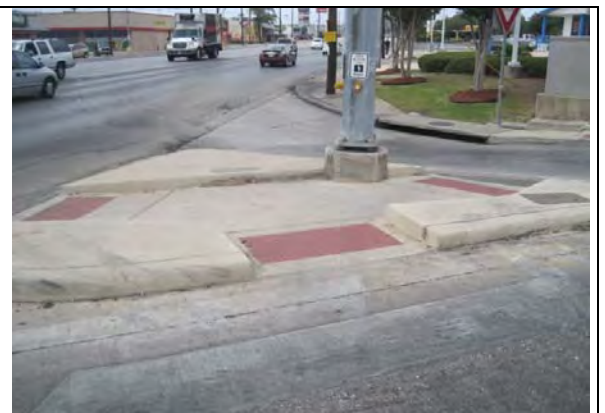
An example of a directional island that provides adequate space for crossing pedestrians, and accommodates wheelchairs.
