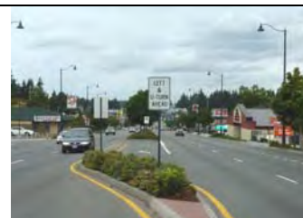
Access management often involves both median installation and driveway consolidation.
