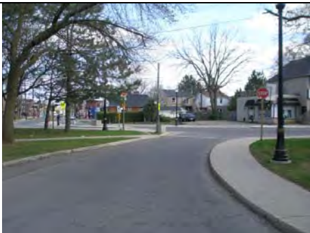
This intersection was designed so that the two roads meet at a 90 degree rather than a skewed angle.
