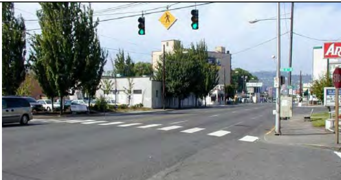
Signal with microwave sensors at intersection . Source: Designing for Pedestrian Safety.
