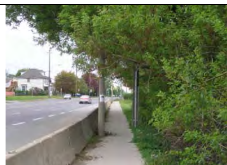
Where there are obstructions within the sidewalk a clear width of at least 1.5 m should be provided.
