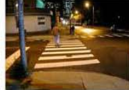
Lighting at Crosswalk
