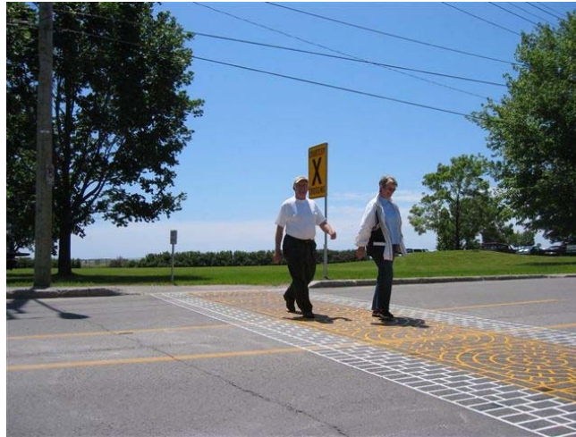
Figure 5: DuraTherm Crosswalk Markings on King Street
