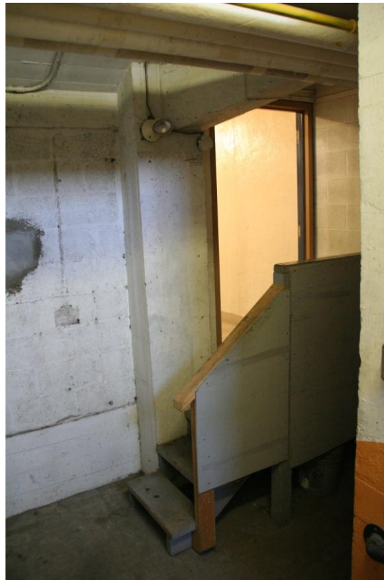
Figure 29: Wooden steps leading from emergency exit hall to women's change room. This doorway constructed in 1974/75. The wooden steps are the exception within the building.
