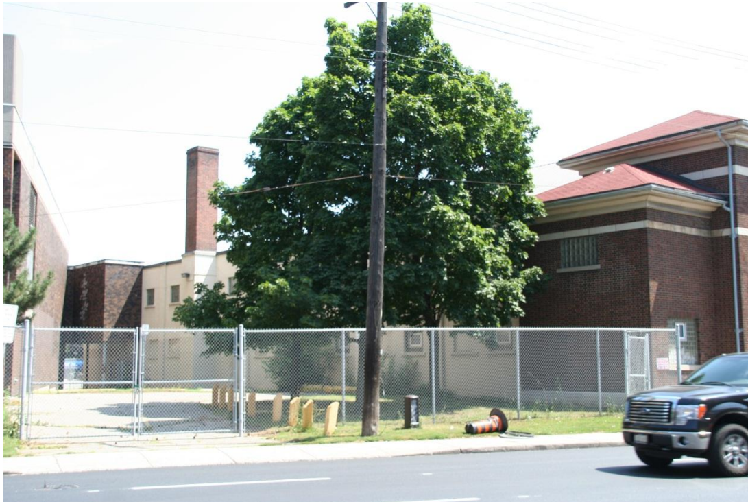
Figure 15: West facade showing brick "bridge" to Scott Park School in rear, behind chimney
