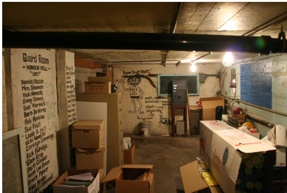
Figure 25: Storage room under pool deck; swimming pool wall on the right, and "Guard Room Honour Roll 1967" graffiti on left.
