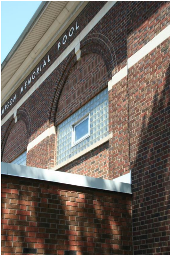
Figure 11: Front (south) Facade detail of brickwork on new addition and original building. Note the decorative brick pattern in the arches.
