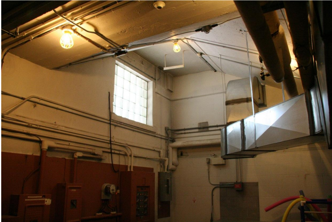
Figure 26: Electrical room showing ground-level windows.
