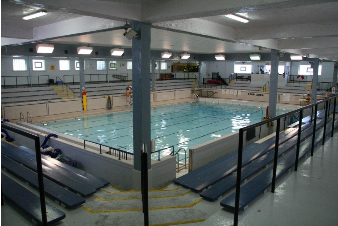
Figure 31: Looking south east to front at King Street and to Balsam Street. Roof columns and judging booth are evident
