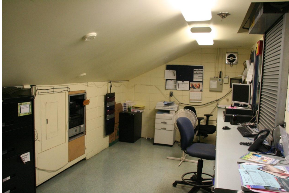
Figure 20: Large office on east side
