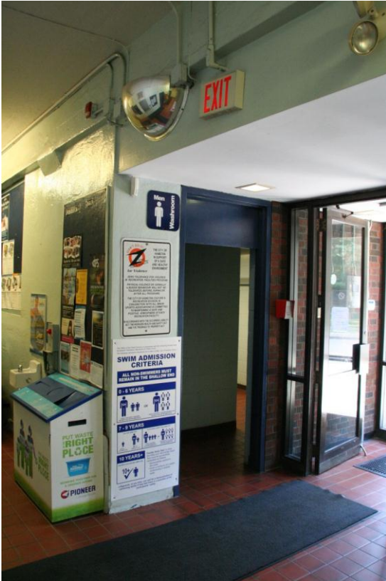
Figure 17: "New" addition showing men's washroom. The original front of the building is the wall on the left.
