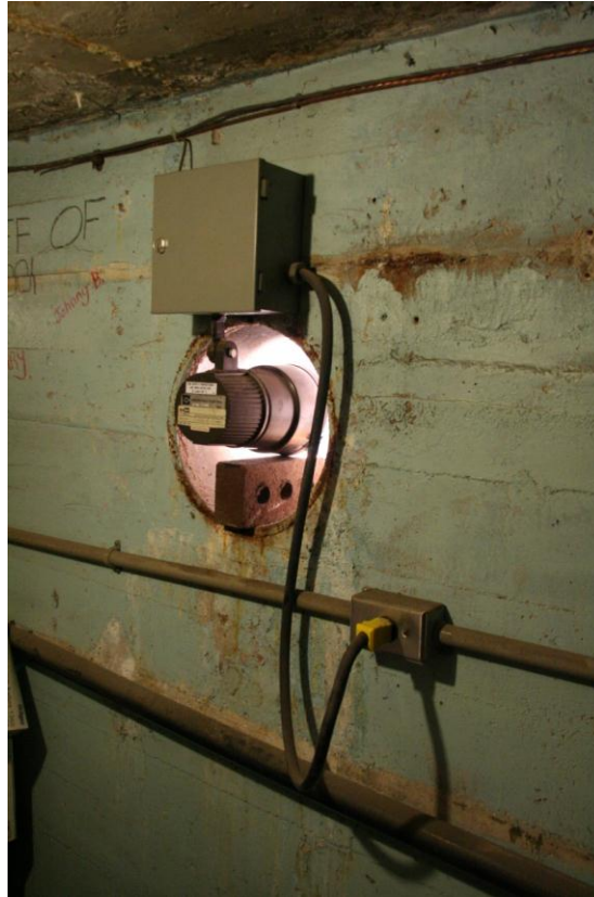
Figure 24: Storage room showing one of the pool's light fixtures on the north end of the pool. The marks of the board forms in the concrete are visible.
