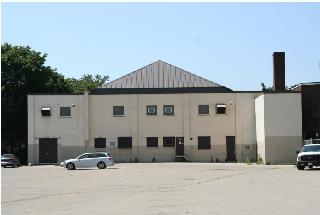
Figure 14: North facade showing hipped roof of skylight, new fire escape extension of right and furnace room chimney
