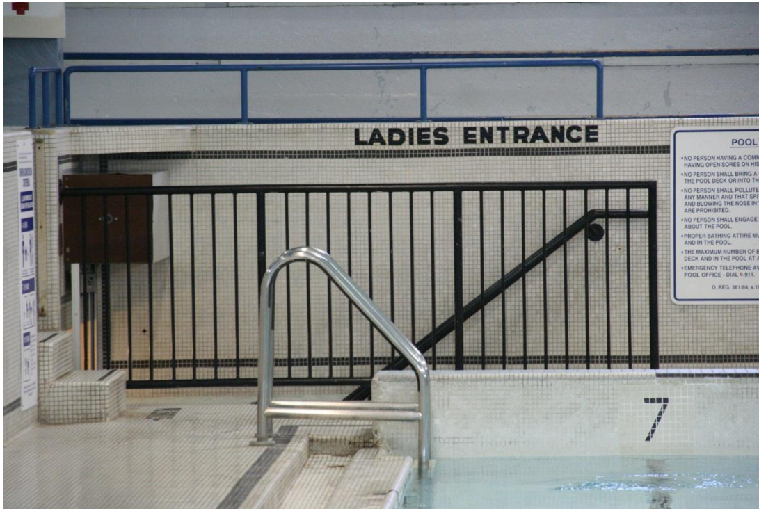
Figure 37: Ladder, barrier tiles, gutter, staircase to women's change room at north west side. The letters are painted
