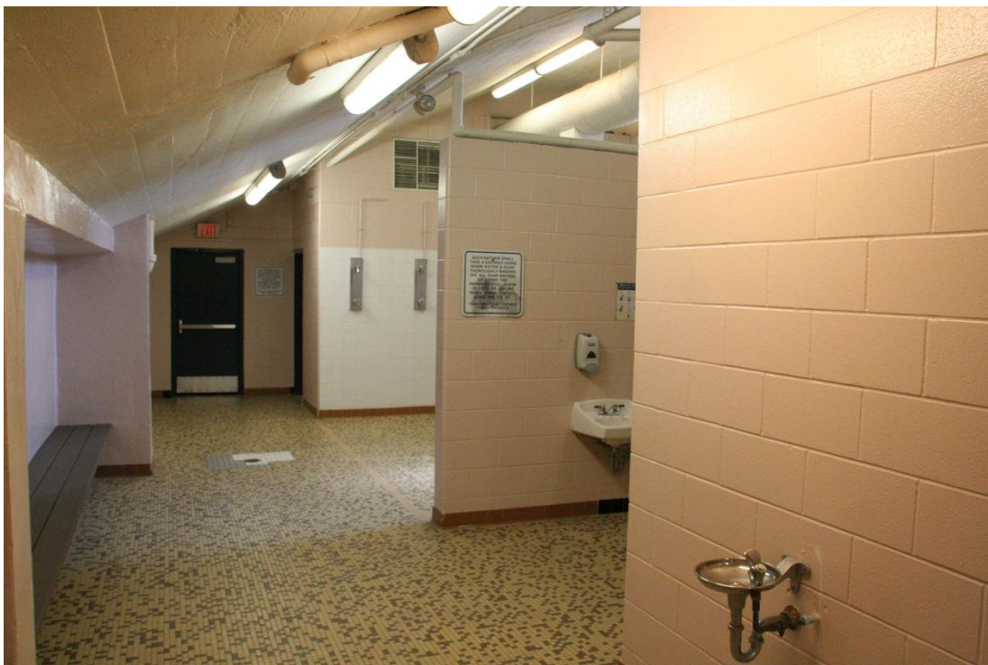
Figure 23: Men's change room looking north showing slope of pool bleachers in ceiling
