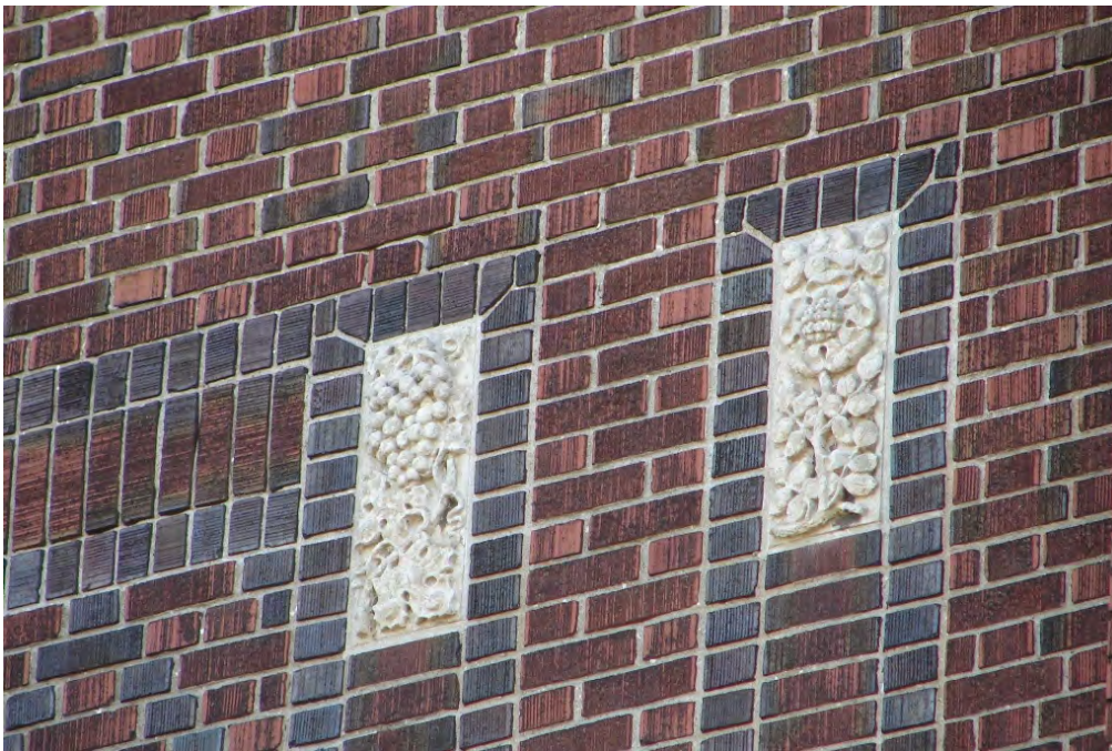
Fig. 51 Carved stone bas-relief panels and brick patterns in blind north elevations of end pavilions
