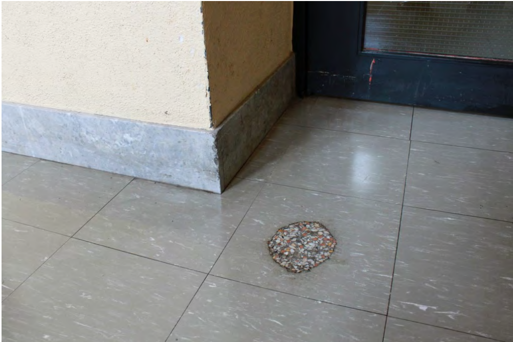
Fig. 131 Terrazzo floor reveal in west end stairway
