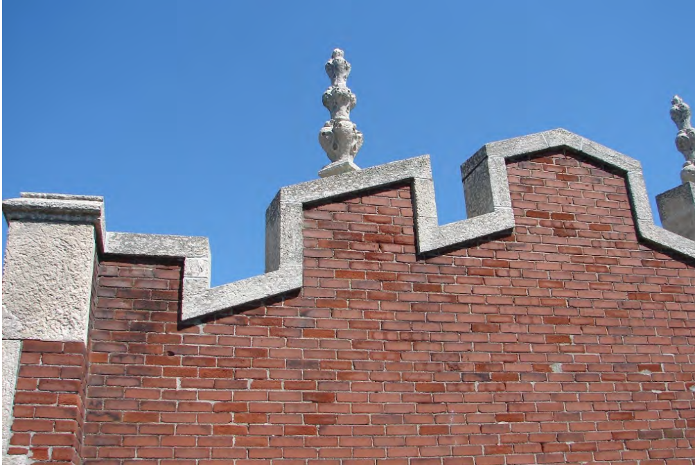
Fig. 68 Detail of parapet, crowned with stone crenellation and finial
