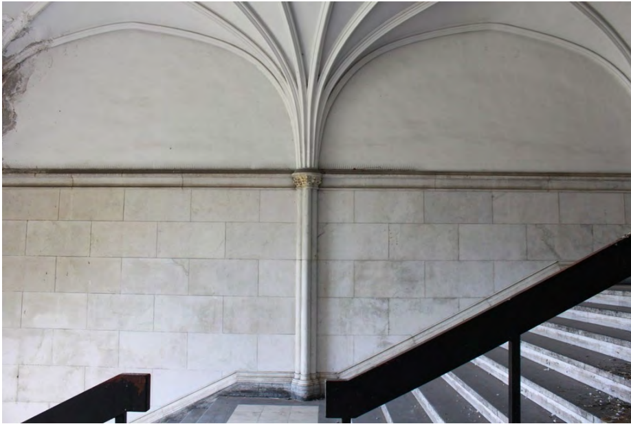
Fig. 43 Entry porch walls in marble wainscotting and fan of vaulted ceiling in stucco plaster
