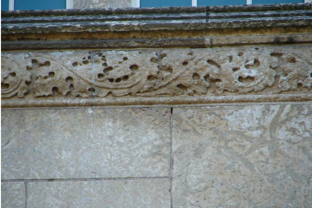
Fig. 35 Carved stone course of acanthus leaves below the cornice of the tower's two-plus-storey front entry porch
