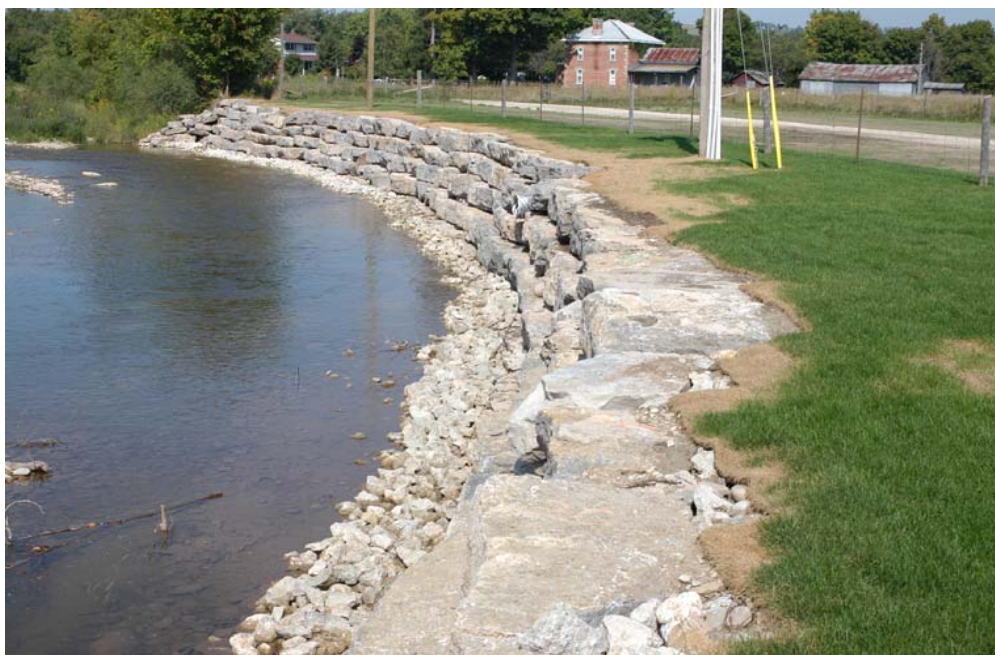
Image E – Armour Stone Seawalls
