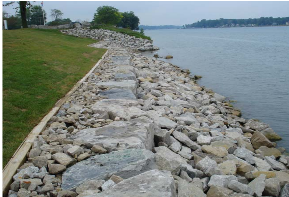
Image A – Rip Rap Revetment with Armour Stone Cap (Similar to concrete cap)
