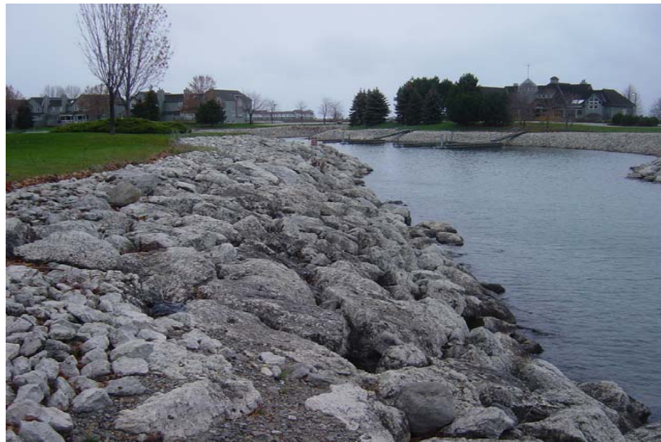
Image B – Armour Stone Revetment
