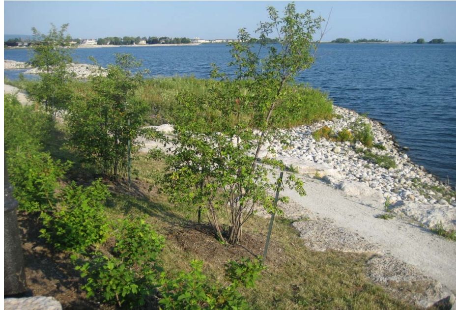
Image C – Cobble Revetment with Aquatic Habitat
