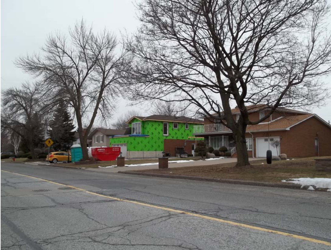
Photo 3: Dwelling addition at 372 Mountain Brow Boulevard
