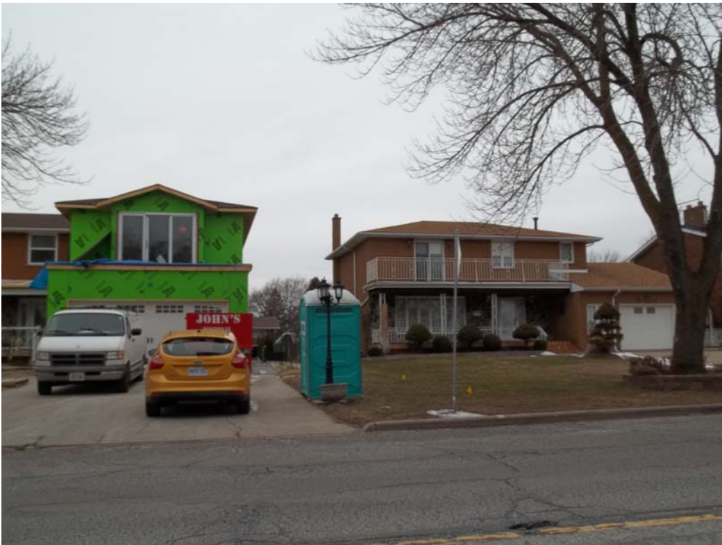
Photo 2: Dwelling addition at 372 Mountain Brow Boulevard
