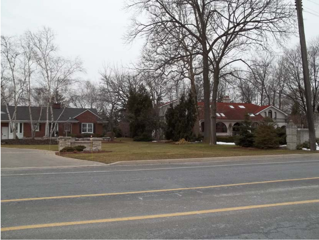
Photo 9: 234 and 224 Mountain Brow Boulevard
