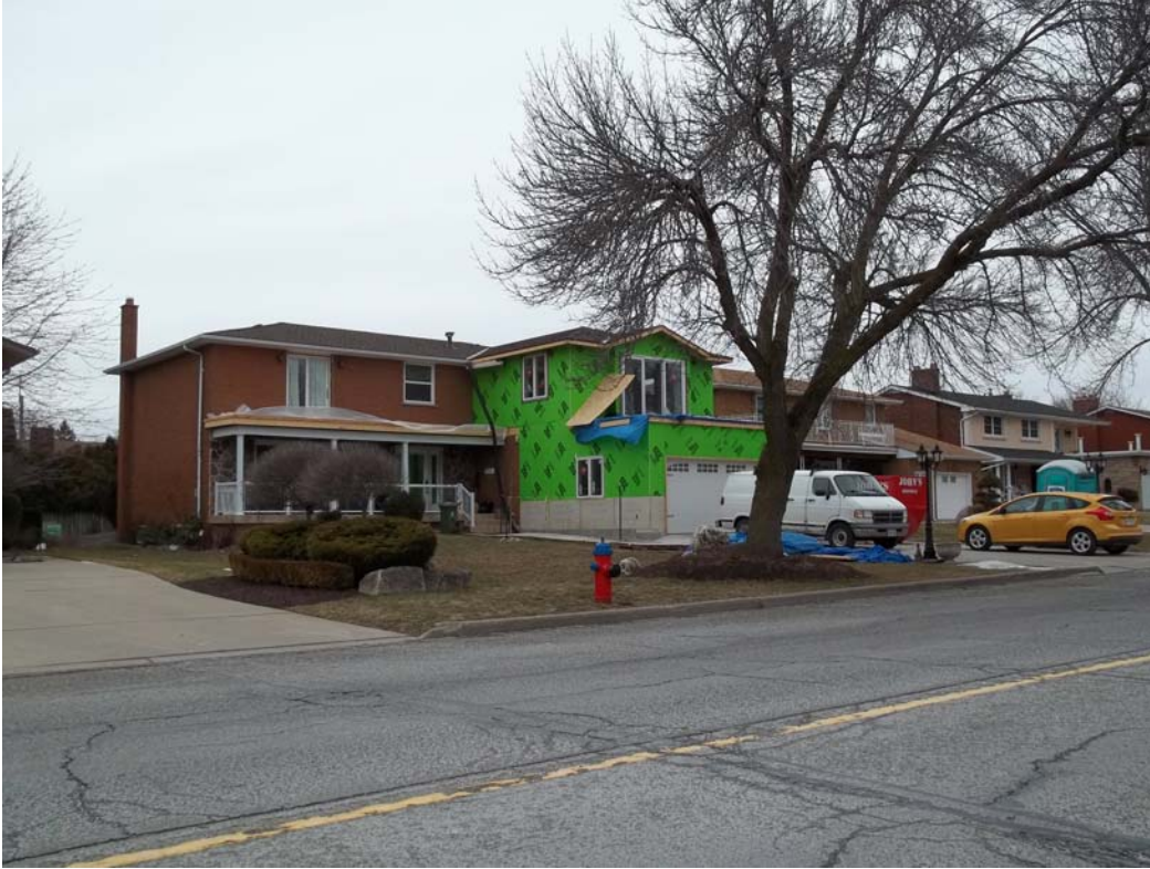
Photo 1: Dwelling addition at 372 Mountain Brow Boulevard
