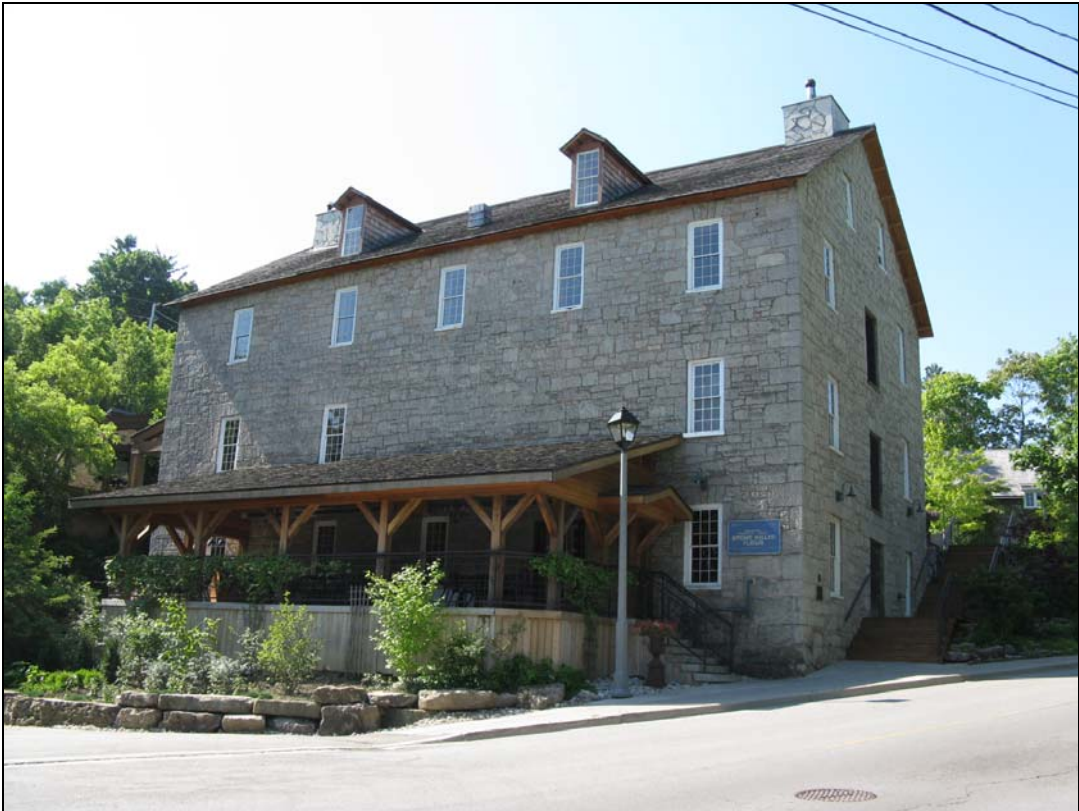
North and West Façades of the Mill Building
