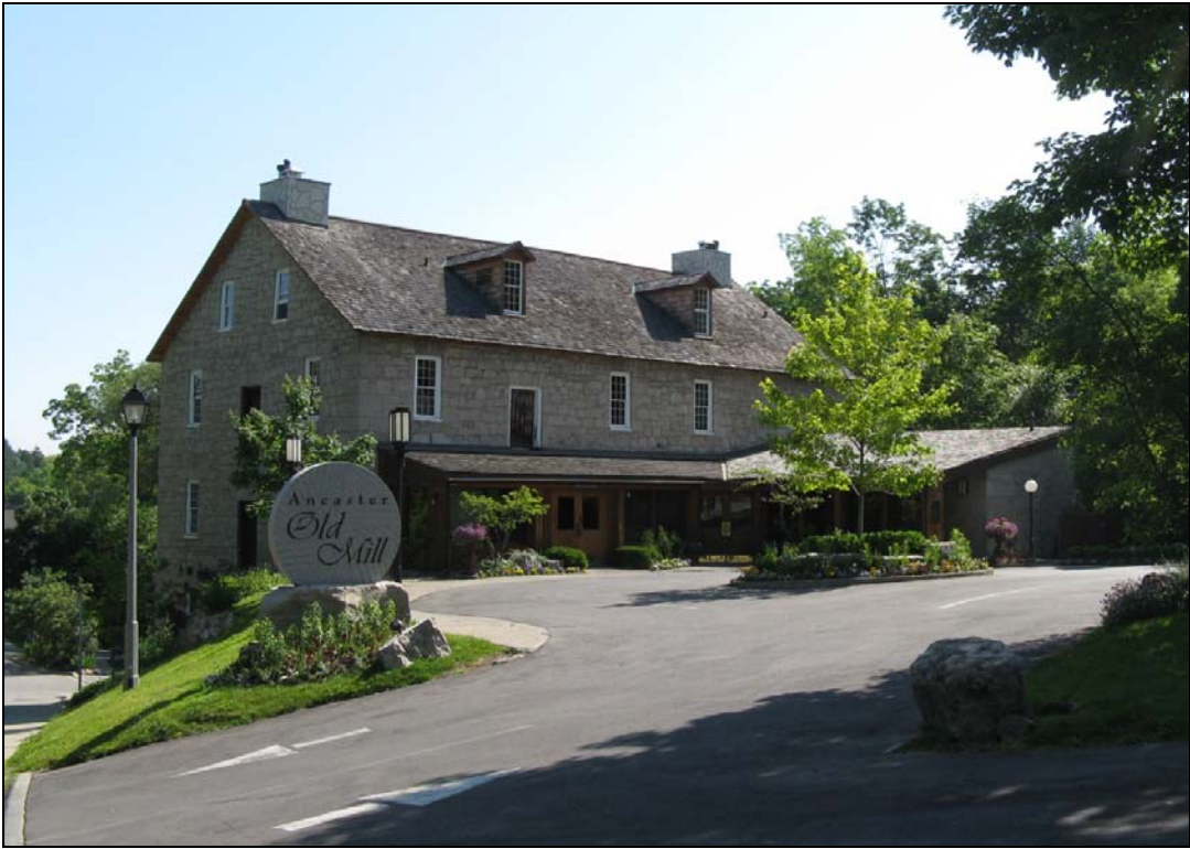
East Façade of Mill Building
