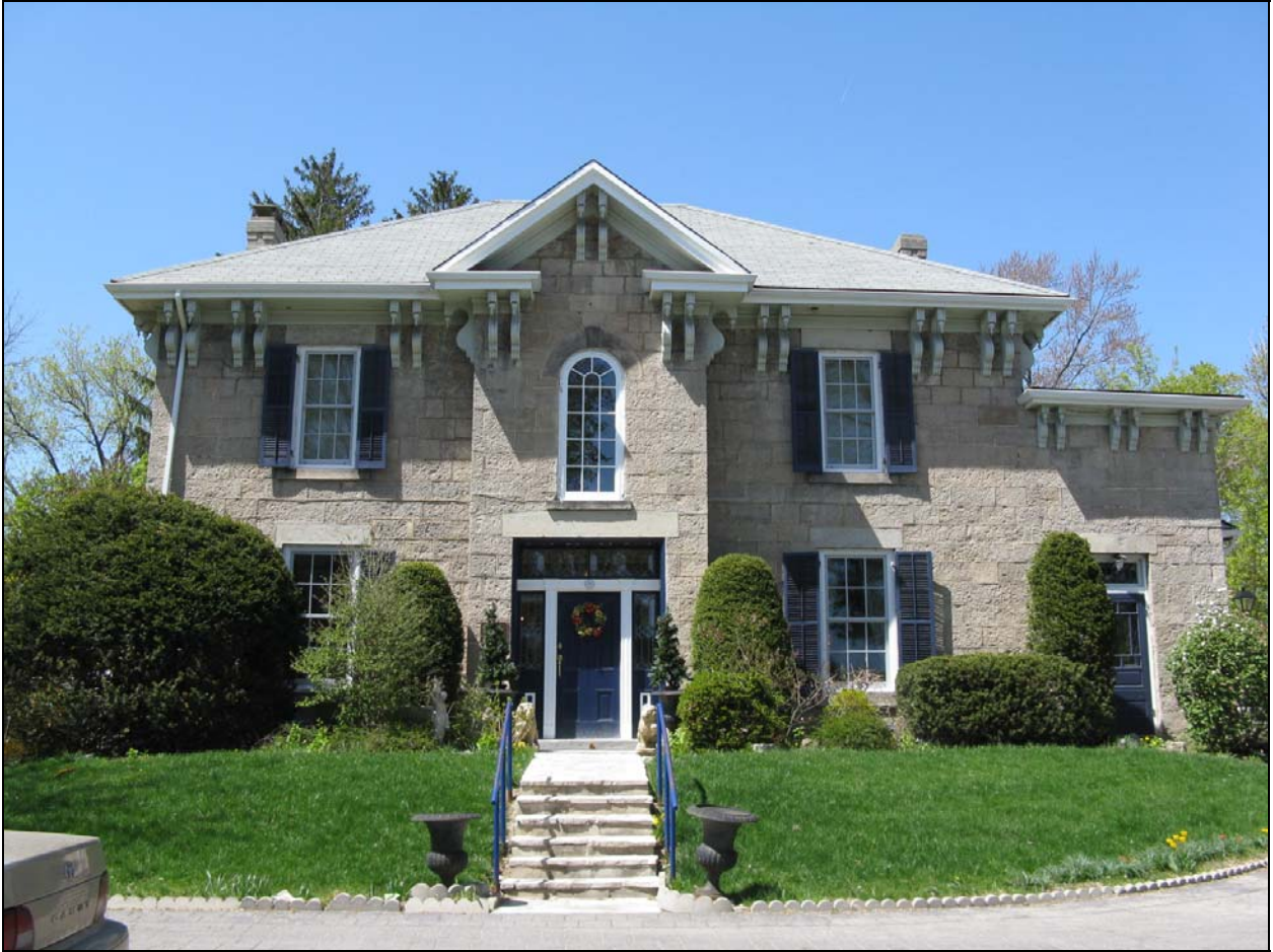
Front (East) Façade
