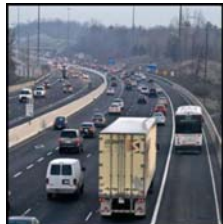
Bus Bypass Shoulders
