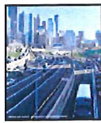
HOV / Transit only bypasses on ramps
