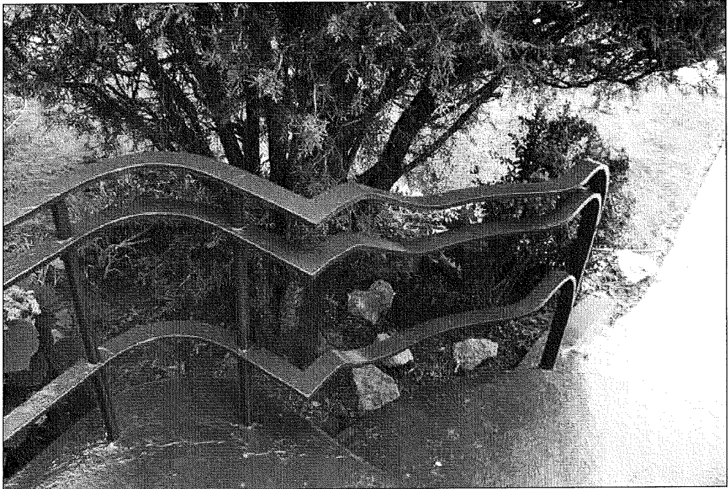
170 Longwood Road North - Curved railings
